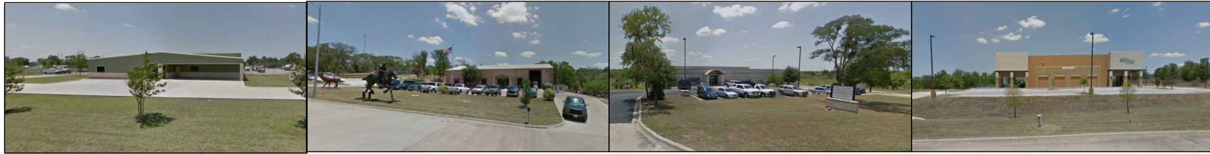
EXISTING BUILDING ON TECHNOLOGY DR
